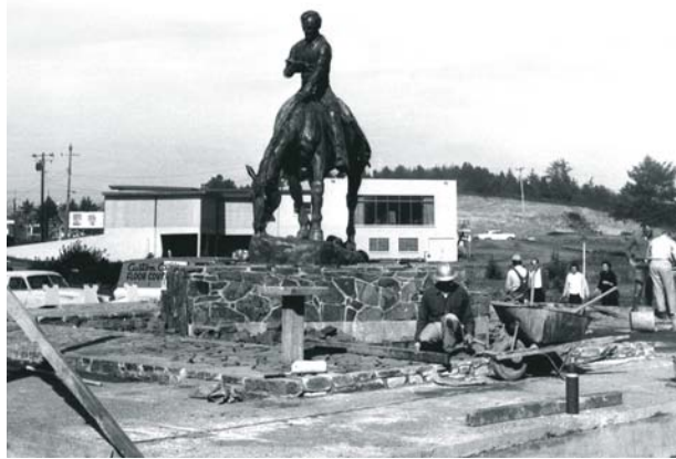
Lincoln Statue 1965 being installed at Kirtsis Park
