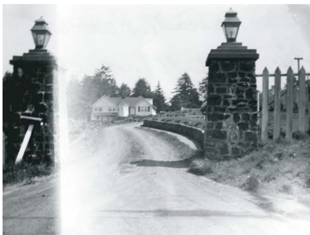
Iris N Ranch in disrepair
