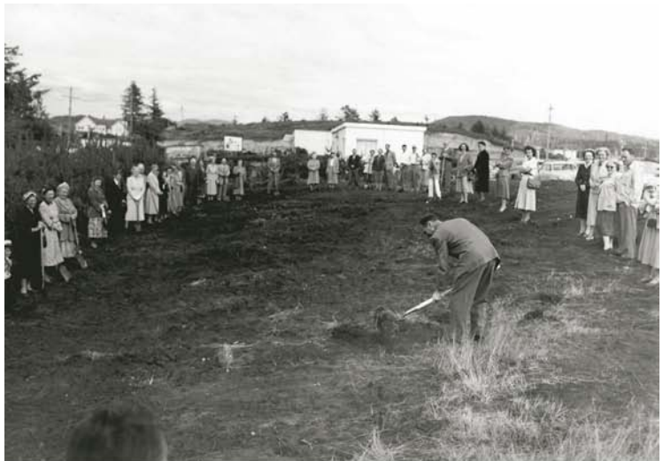
Congregational Church groundbreaking
