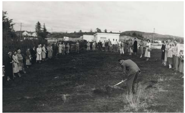
Congregational Church groundbreaking
