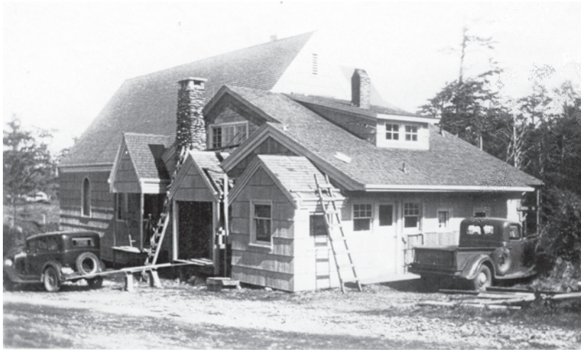
Bateman Mortuary under construction
