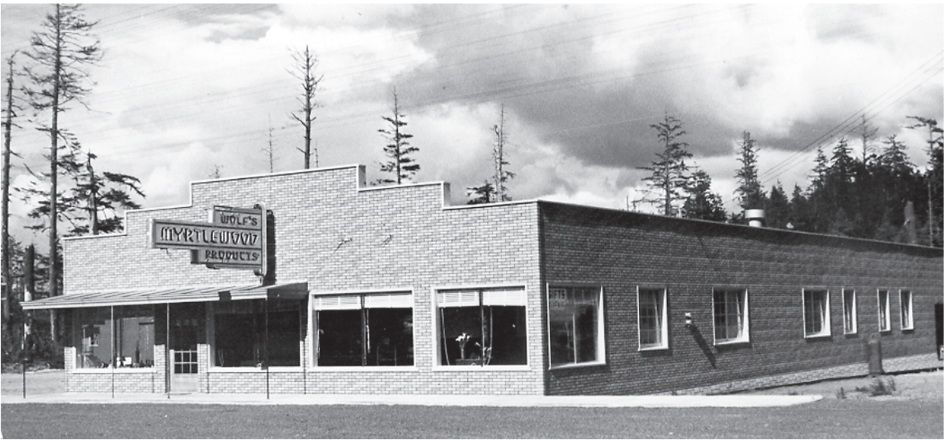
Myrtlewood Products Plant
