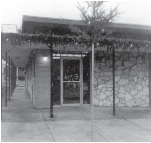
Telephone Company building
