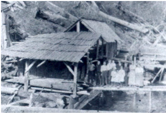
Holton Logging Operation
