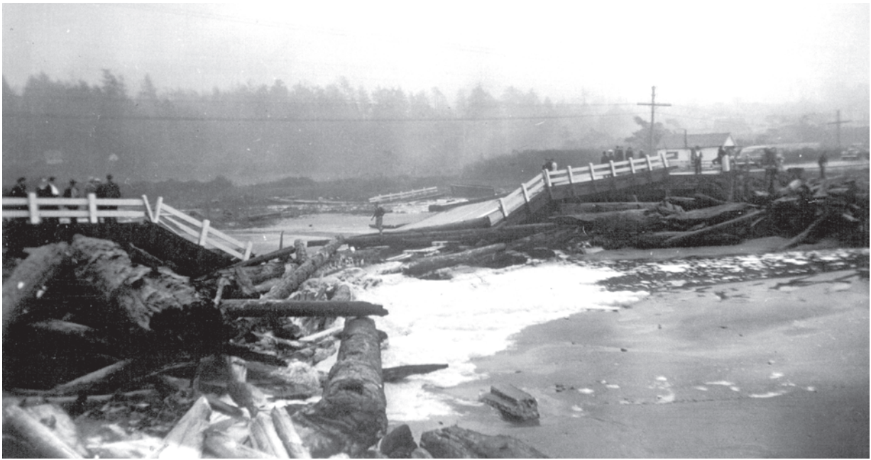
D River Bridge damaged by storm
