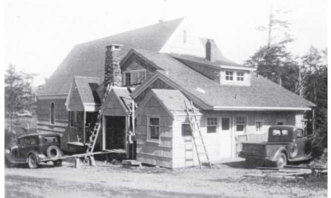
Bateman Mortuary, now Pacific view, under construction
