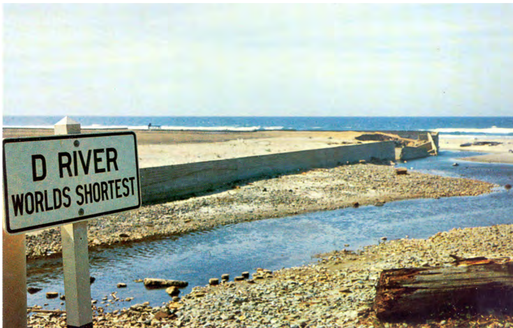
Reinforced channel for D River
