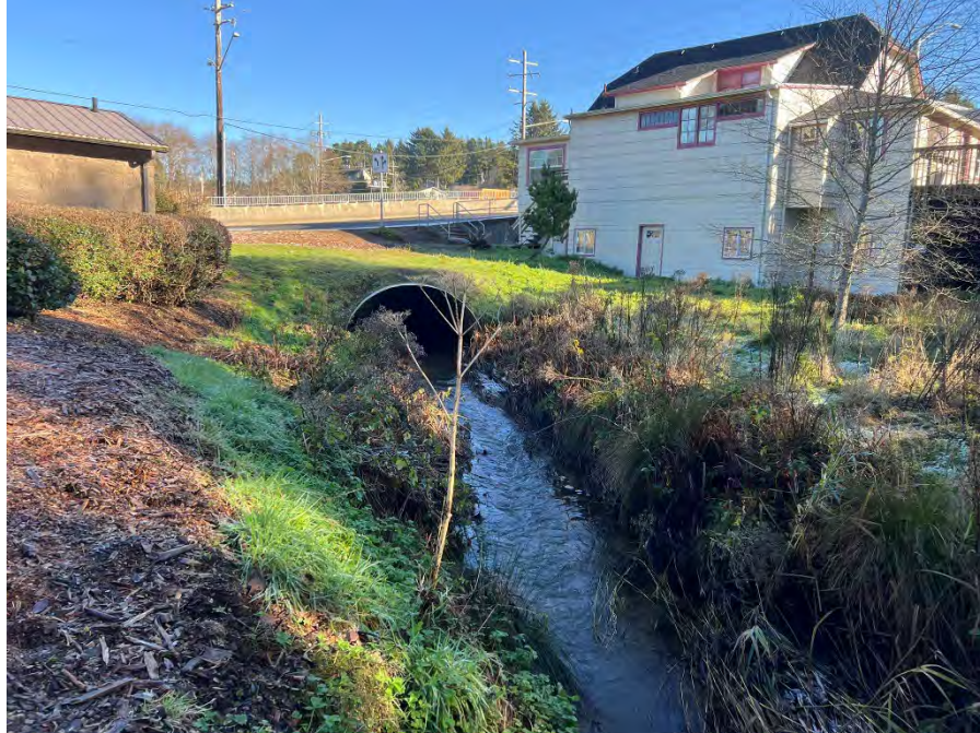
Photo 15. Baldy Creek and culvert, facing northeast. Photo taken December 3, 2024.
