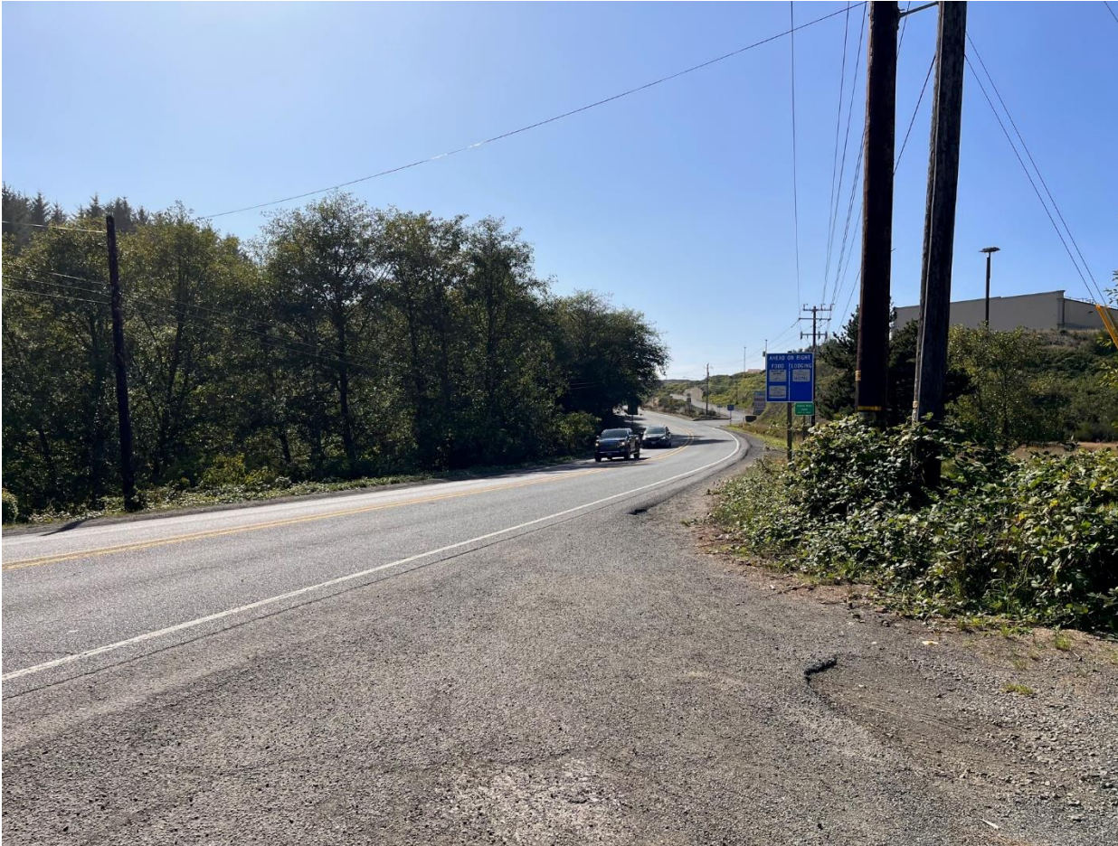
Figure 6. Existing view from the residential driveway facing toward northbound US 101. The figure shows that the full width of the Lighthouse Square access is visible; trimming of vegetation along the curve and relocation of the tourist information sign would be beneficial in further improving these views due to the slight incline toward the southwest.
