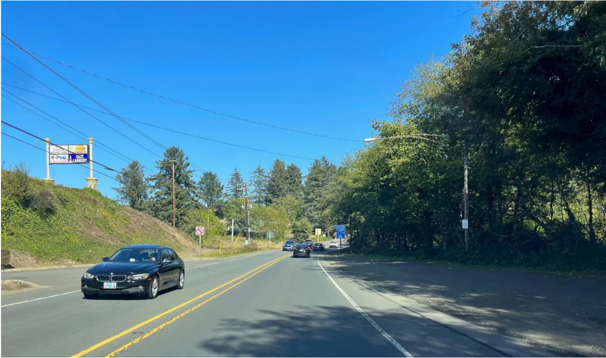
Figure 8. Stopping sight distance from 500' south of the access. The access is visible, but partially blocked by the tourist information sign.
