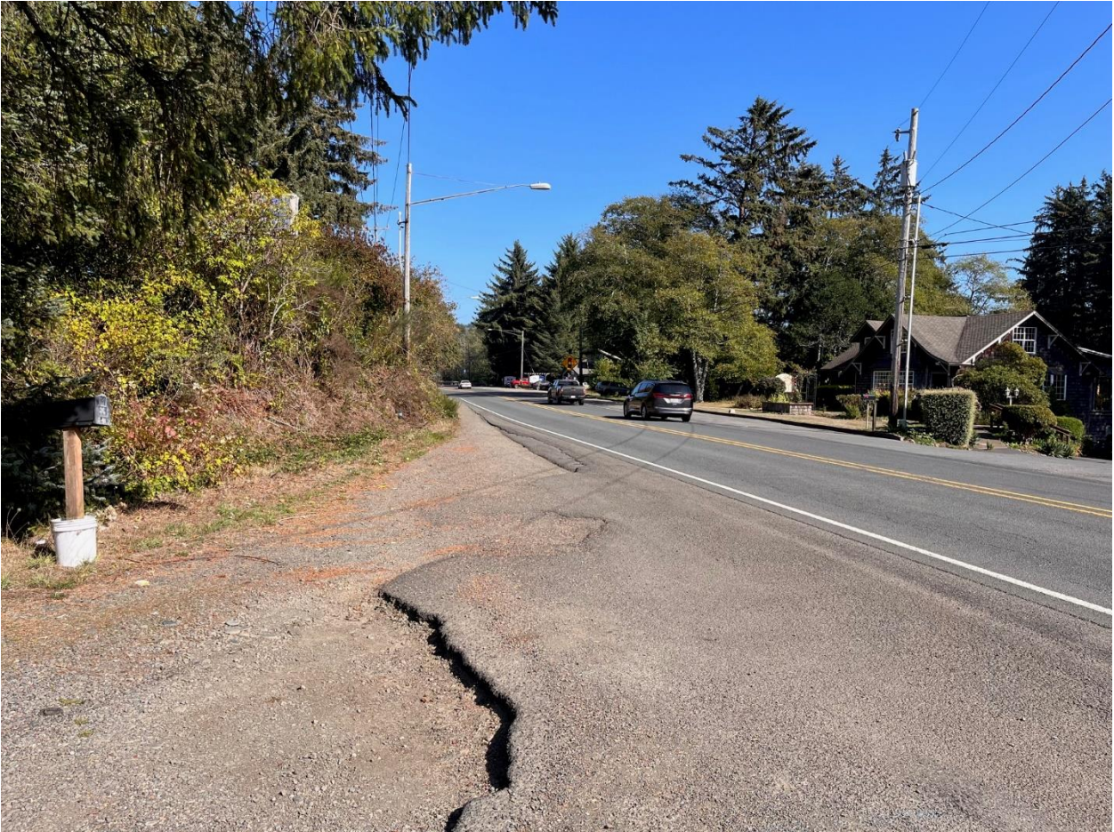
Figure 7. Existing view of southbound US 101. The shows that the embankment limits existing sight lines, and minor trimming and/or grading could be beneficial in further improving these views.
