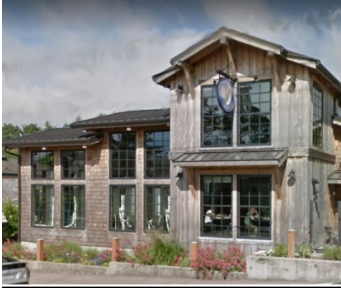
Variations in wood siding, concrete base, and metal roof and awnings.
