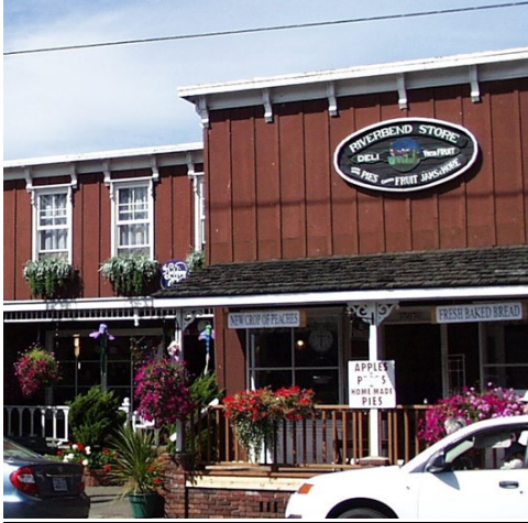
Flat roof with projecting cornice of a different color.
