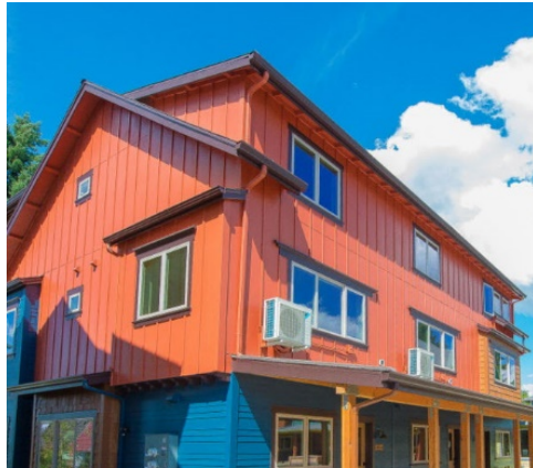
Pitched roof with attached shed roof.
