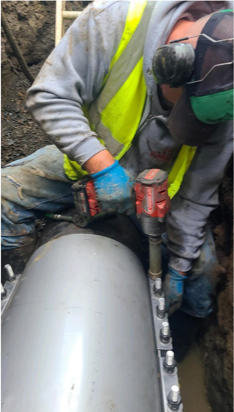
Figure 2 Installing the repair band
