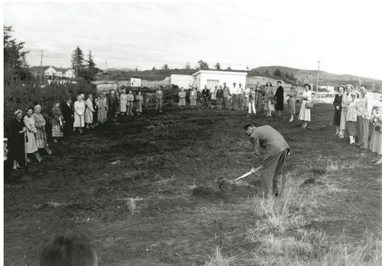
Congregational Church groundbreaking
