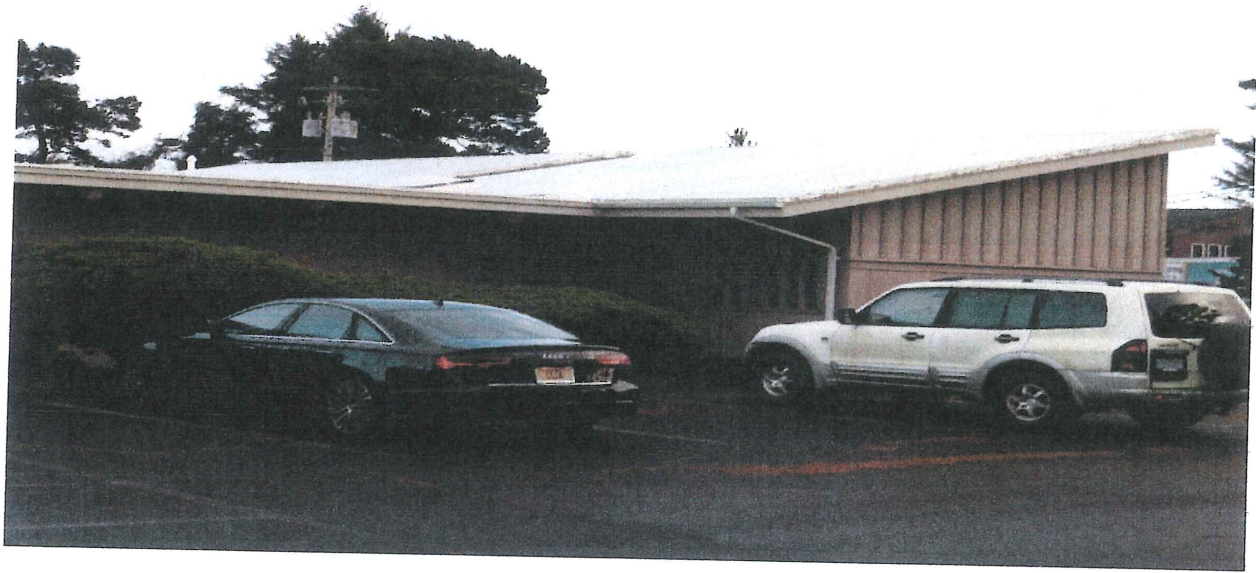
Below is a close up of this roof area.
