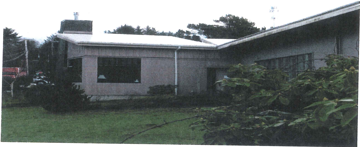
Street view of east section of the building including roof
