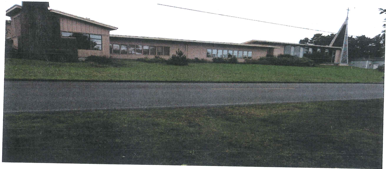
View from 25 th Street
