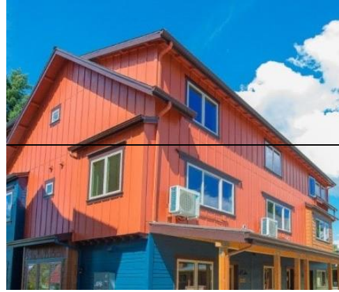
Pitched roof with attached shed roof.
