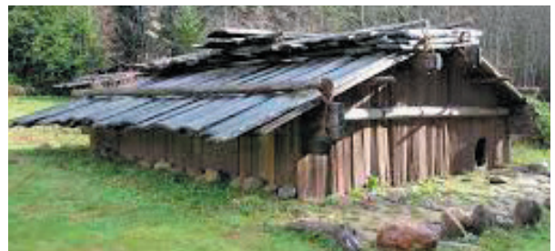
Native American plank house
