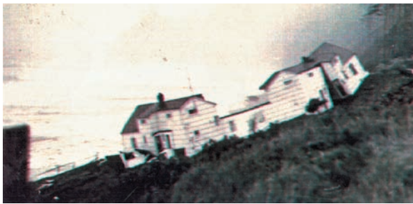
Seagull Apartments beginning to slide off the hill.
