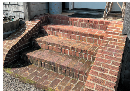
Brickwork at front entrance to Roads End Apartments, 2023
