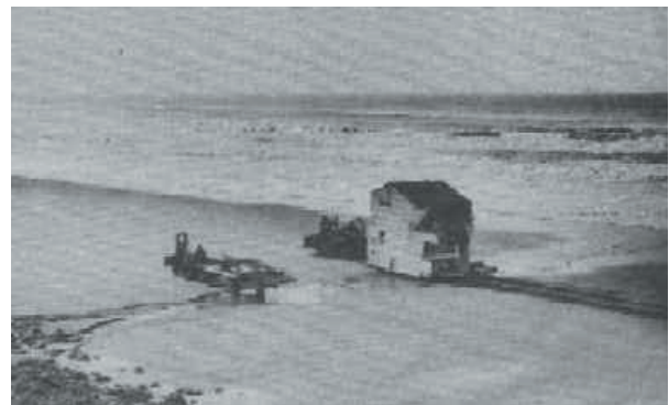
Seagull Apartments being hauled down the beach.
