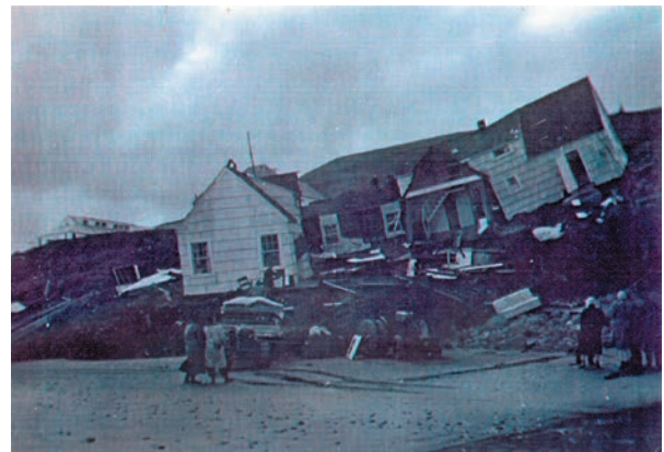
Seagull Apartments after landslide
