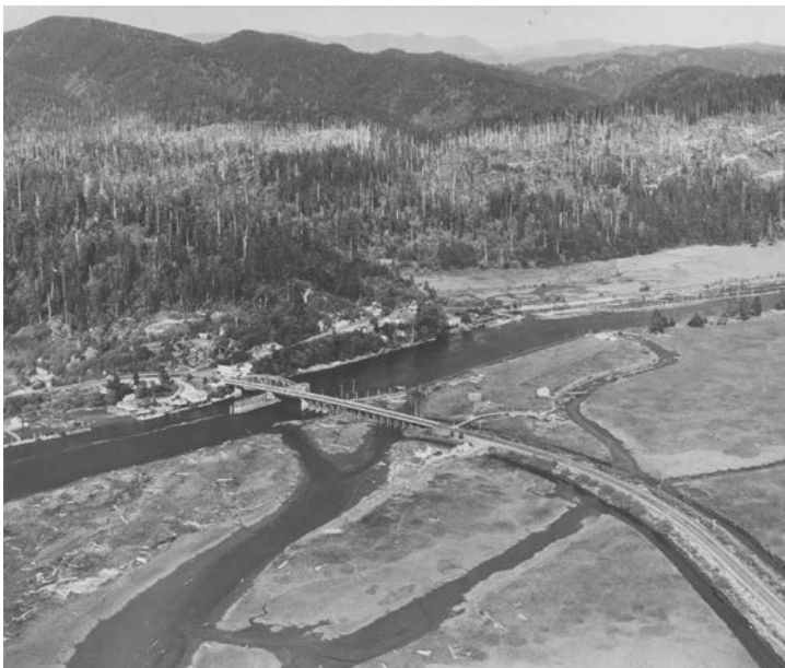
Kernville Bridge over Siletz River,, built 1924
