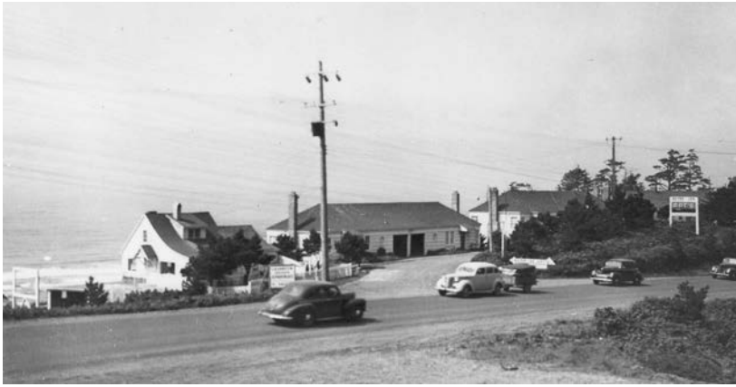
Ester Lee Apartments, looking west from Highway 101 circa 1943
