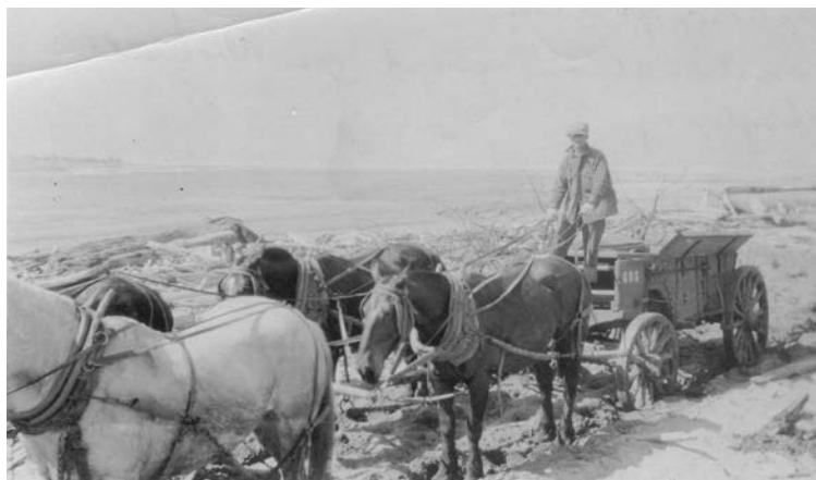
Building the Coast Highway
