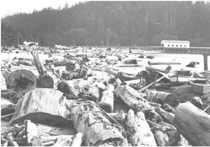
Bridge over Schooner Creek, built 1927
