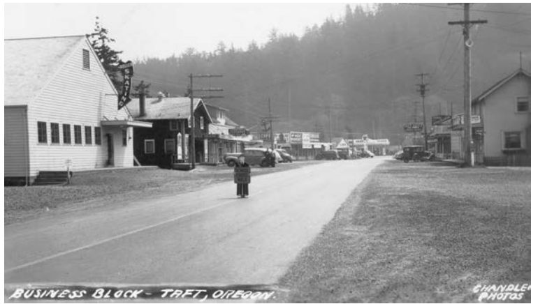
Looking south on Coast Highway in Taft. On the left: skating rink, Lincoln Theater, and Pines Hotel
