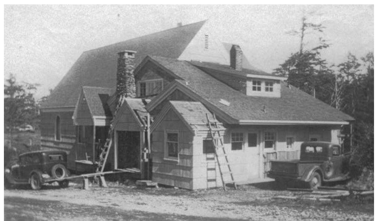
Bateman Mortuary under construction
