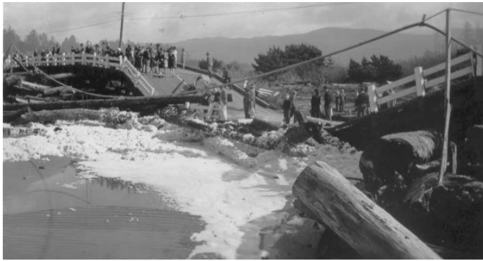
Debris from 1941 storm, top; D River Bridge washed out in 1941 storm, bottom
