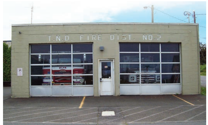
Delake TND Fire Station
