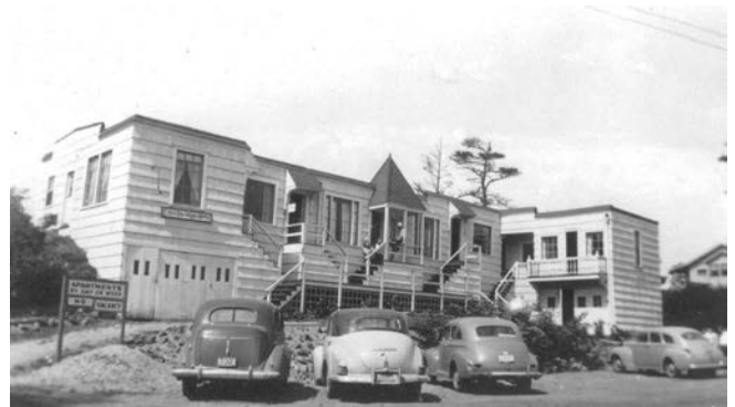
Casa Del Mar after conversion to apartments in the late 1940s
