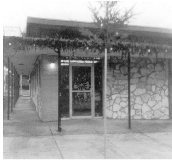
Telephone Company building
