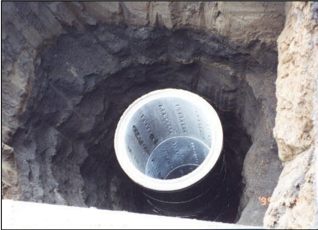
Commercial drywell Installation in Portland, OR
