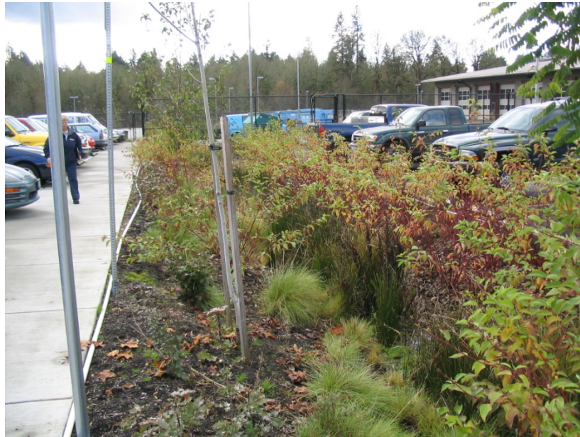
Biofiltration Swale at Clean Water Services Field Operations Building in Hillsboro, Oregon
