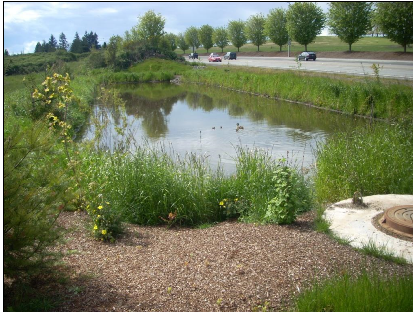
Combination Wet/Detention pond adjacent to Kuebler Boulevard in Salem, Oregon.
