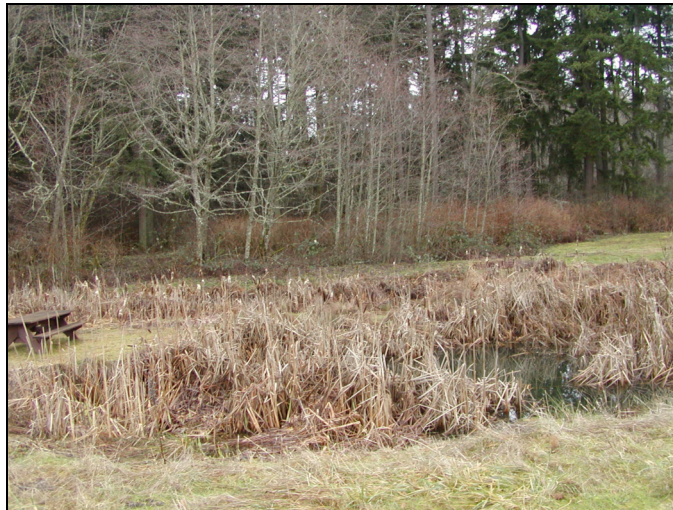
Constructed stormwater wetland in Olympia, Washington
