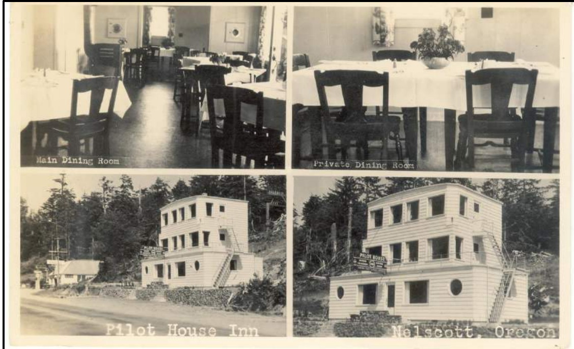
Figure 26 – The modern metal awning at Nelscott’s Foon Hing Yuen building (see here c.1946 as Pilot House Inn) presents another mural opportunity. From the Collections of the North Lincoln County Historical Museum and Society, Lincoln City, Oregon.
