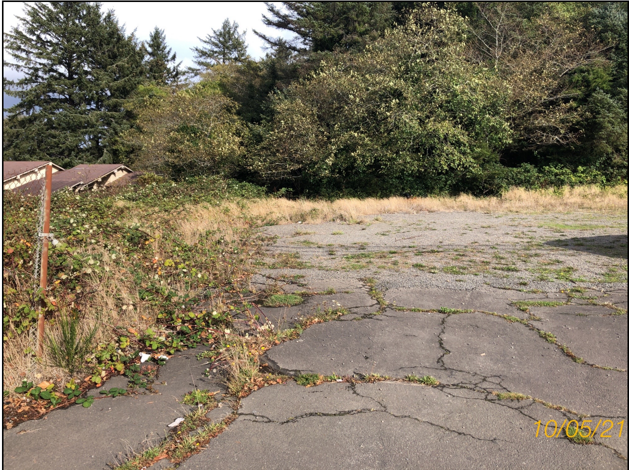
Photo 1: Looking east at the north end of the western-most lot.
