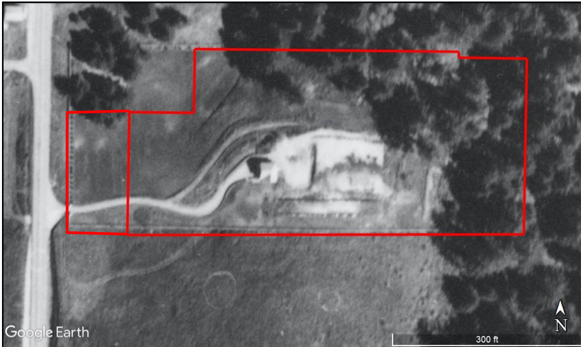
Figure 4: 1939 – The Estate appears to still be under construction. The main house and retaining walls are visible, but no buildings have been constructed in the area east of the main house which appears to be graded.
