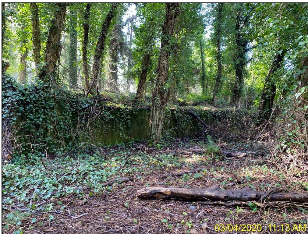
Photo 2: Upper area, terraced with retaining walls (near TP-5).
