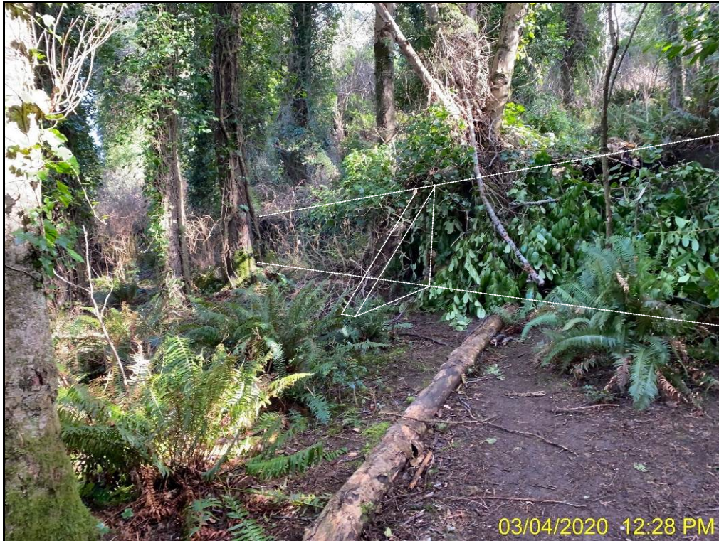
Photo 9: Lower driveway area with buttressed retaining wall covered in vegetation.
