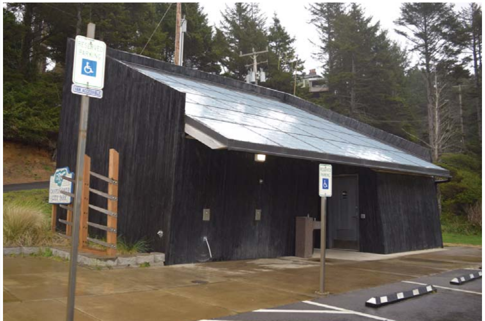
Canyon Drive Restroom
